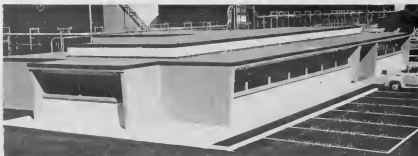
NEW QUARTERS for Zone 1, occupied Nov. 26, are shown here. It is located just behind the Cracking Plant office and houses the mechanical crafts operating in the area.
